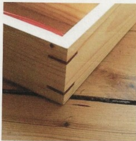
Photo 6 - Spline placed 90 degrees to the Miter
